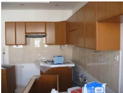
The new kitchen in progress
